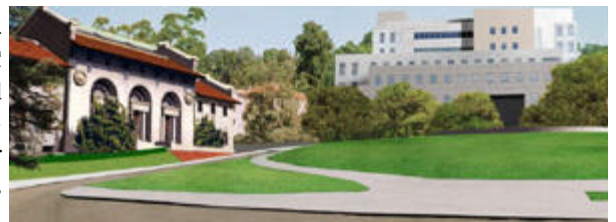
Front view of new Stanley Hall
